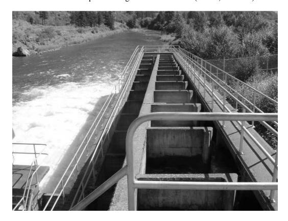
**Figure 2.1.** A photo of the vertical slot fishway at the Seton river hydropower facility used to facilitate upstream migration of salmonids (source, L.B. Pon).
