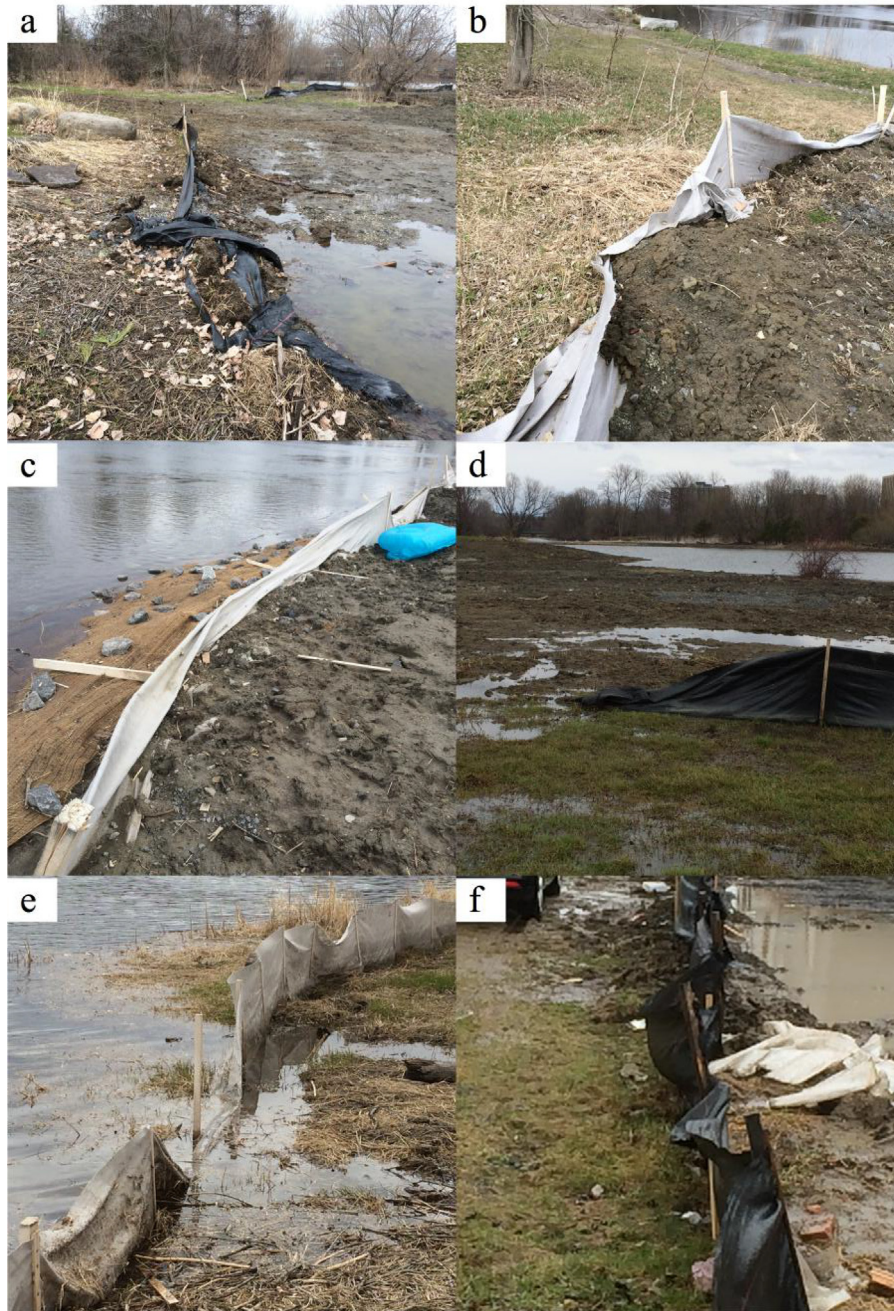
Fig. 1. Common problems with silt fence installation and maintenance observed in Ottawa, Ontario, Canada. All of these problems can lead to unnecessary silt deposition into aquatic ecosystems. a) Fencing that has fallen over with broken wooden support poles, b) Sediment piled upon and over silt fencing, c) Wooden support poles removed causing fence to collapse, d) Insufficient fencing, e and f) Loose and ripped fencing.
