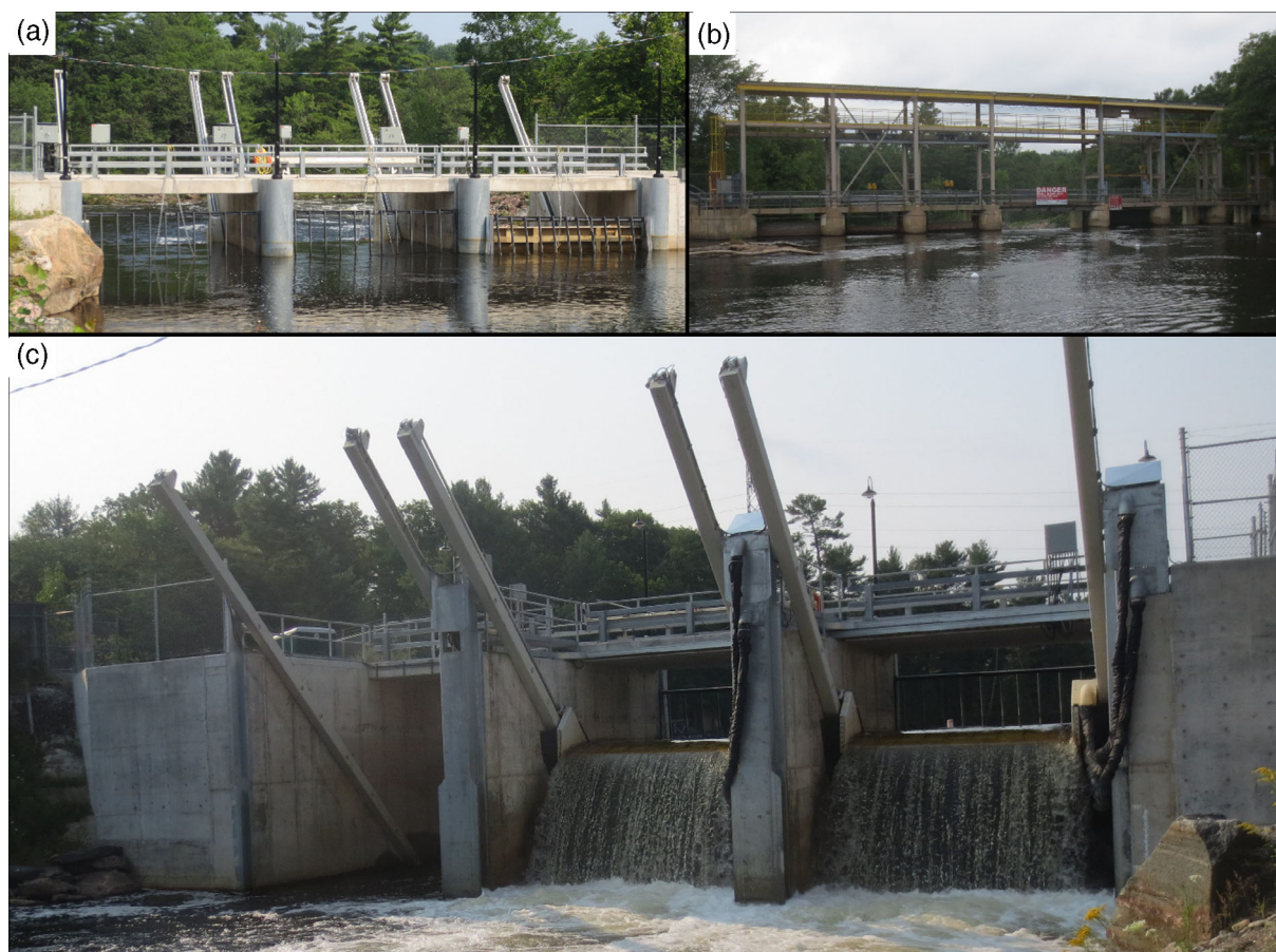
FIGURE 2 (a) Very Low Head turbines at Wasdell Falls looking downstream. (b) Water control dam on East side of island from VLH turbines. (c) VLH turbines looking from downstream to upstream [Color figure can be viewed at wileyonlinelibrary.com ]
