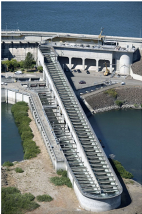
Fig. 2 The submerged east orifice fishway at the Dalles Dam on the Columbia River, USA. Photo credit: USGS
