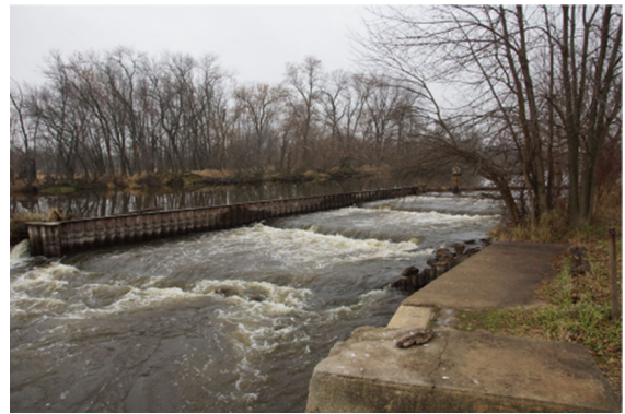
Fig. 5 The three step plunge pool Eureka Dam fishway on the Upper Fox River, Wisconsin, USA. Photo credit: Wisconsin DNR
