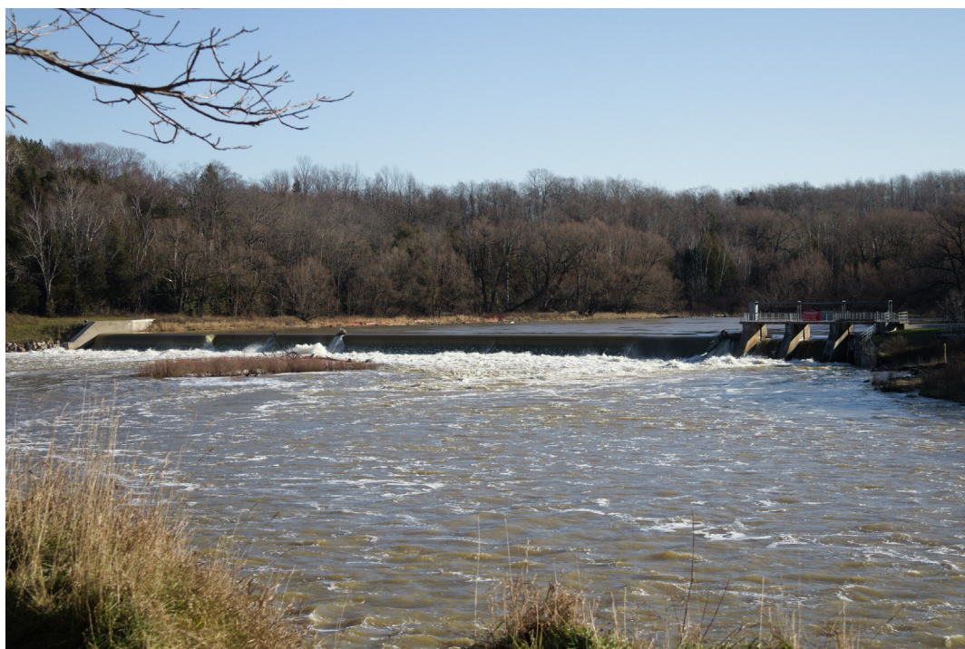
Fig. 1. The rehabilitated sea lamprey barrier named Denny's Dam on the Saugeen River in Saugeen Ojibway Nation Territory, photo taken in 2021.
