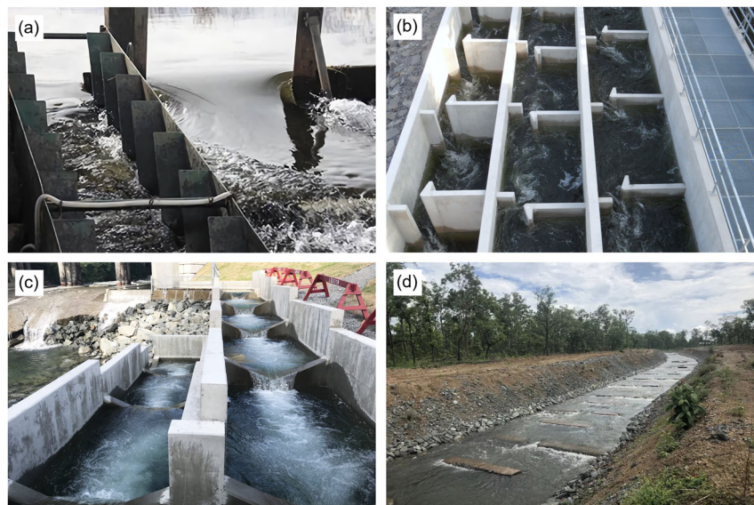
Figure 13. Different types of fishways. (a) Denil fishway for Arctic grayling in the Big Hole River watershed in Montana, Canada (source: Montana State University, photo by Matt Blank, 2015; https://www.montana.edu/eco hydraulics/research/ ). (b) Vertical-slot fishway in the Mosel River in Koblenz, Germany (source: The Federal Waterways Engineering and Research Institute (BAW); https://www.baw.de/en/die_baw/wasserbau/umwelt/umwelt.html ). (c) Pool-weir fishway for migrating pink and coho salmon to spawning grounds in Anderson Creek, Canada (source: McElhanney Company; https://www.mcelhanney.com/project/anderson-creek-fishway/ ). (d) Nature-based bypass fishway beside the Se San River of Cambodia (source: the Xinhua News Agency; https://new.qq.com/rain/a/20191026A099LC00 ).
